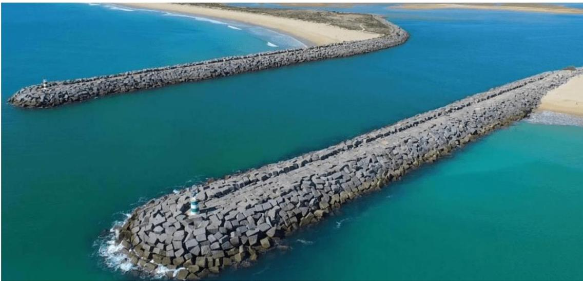
Figure 4. Usual configuration of a rubble mound breakwater in Ria Alvor, Portimão [12].
