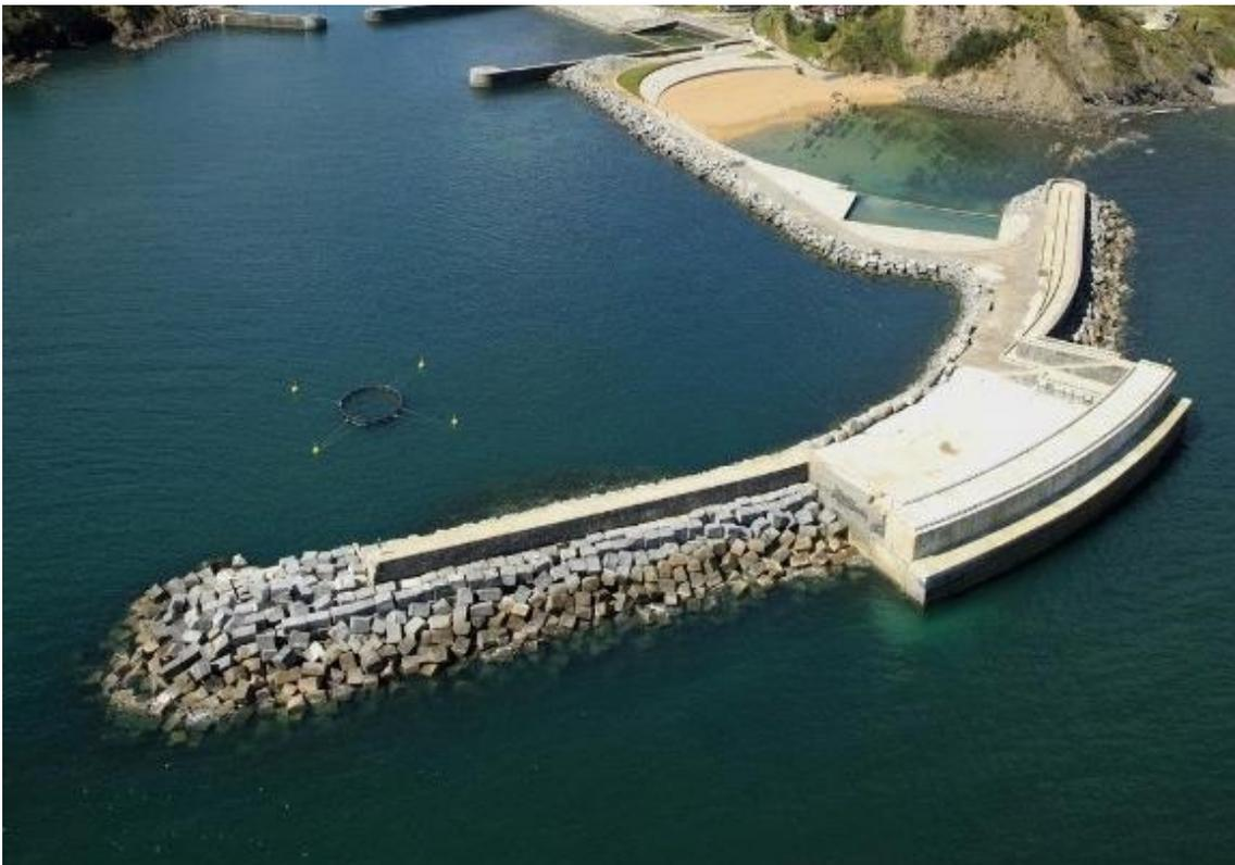
Figure 13. Mutriku OWC breakwater integration [23].
