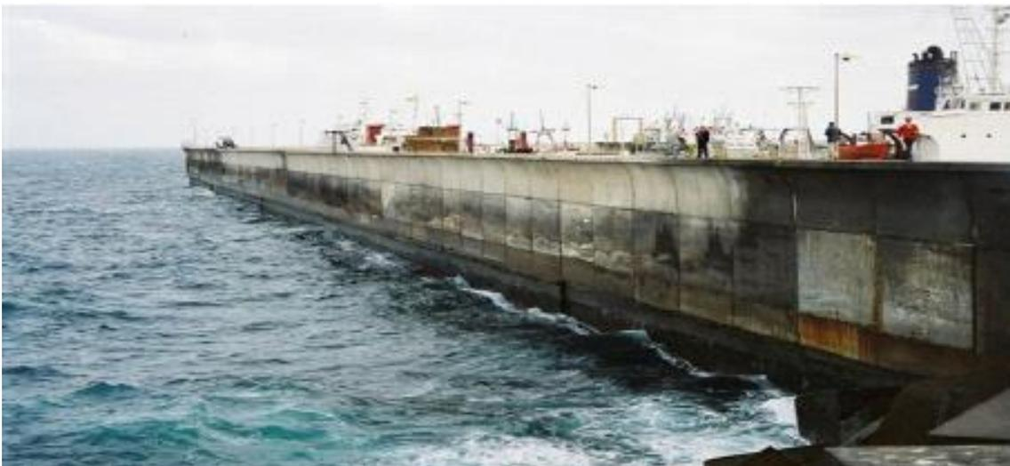
Figure 6. Example of a modern large vertical breakwater [13].
