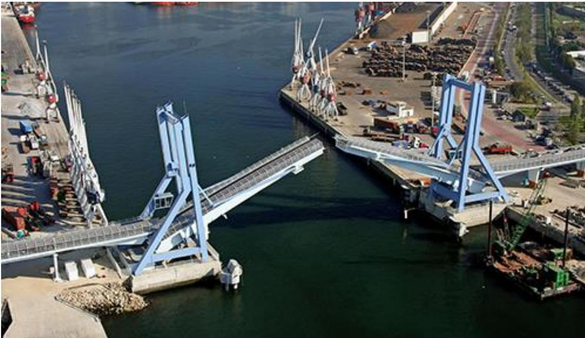
Figure 25. Moveable bridge across the Leça River in the Port of Leixões [45].
