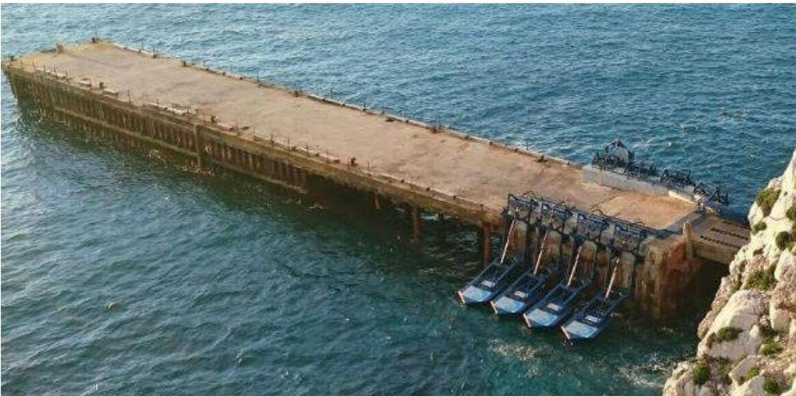
Figure 16. EWP WECs placed in the Gibraltar old ammunition jetty [27].
