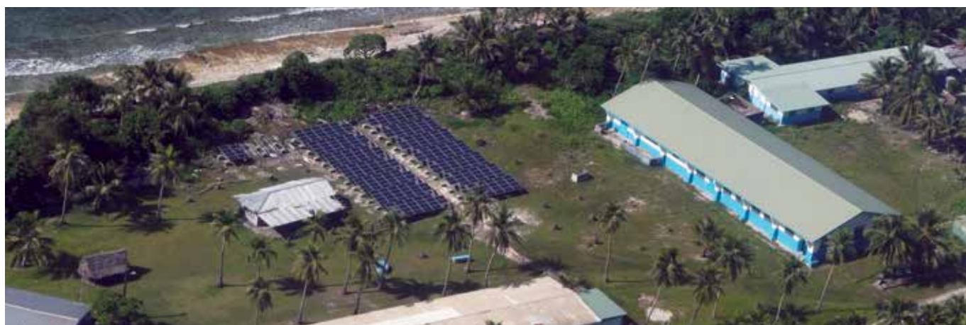
Figure 60: 60 kW solar mini-grid in Ulithi high-school, Yap State, FSM
