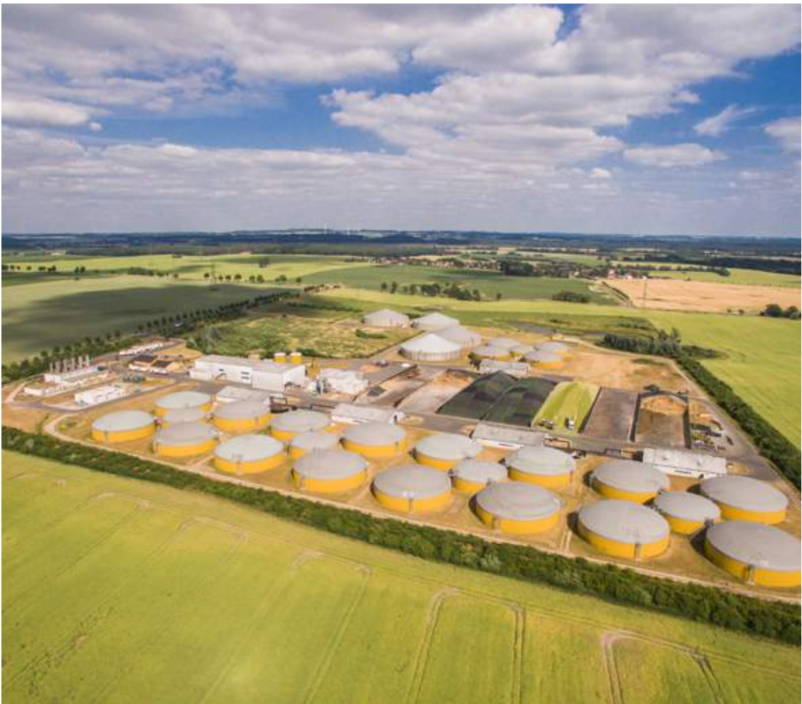
Large biogas plant in Germany.
