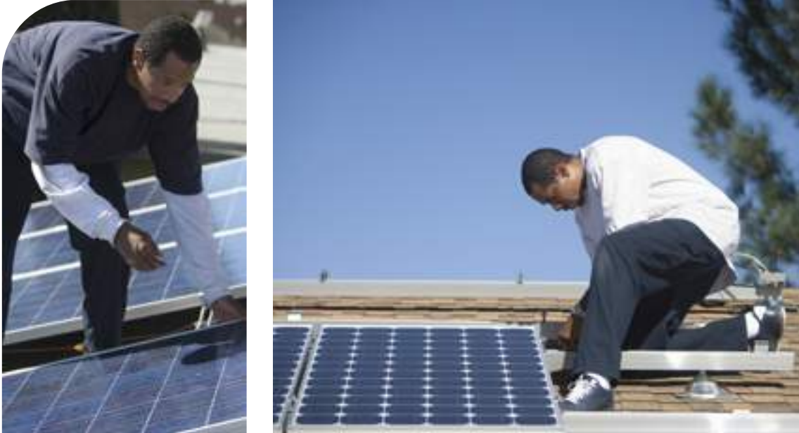
Workers installing solar panels, Shutterstock
