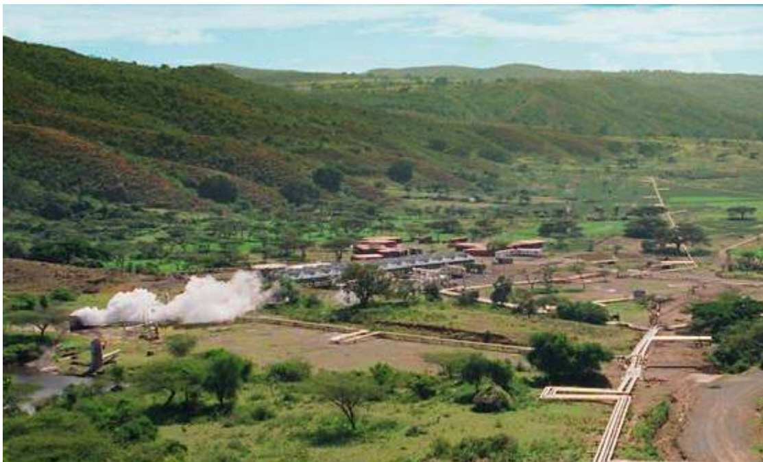
Aluto Langano Geothermal Power Plant, Ethiopia. Photograph: CSI Energy Group
