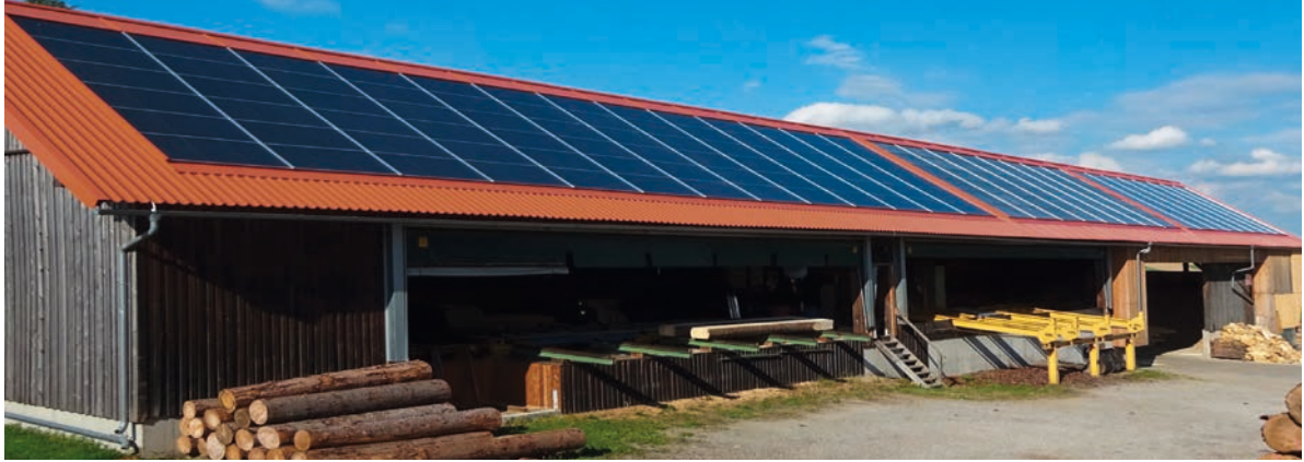
Solar wood chip drying with air collectors, Austria Photo: Austria Solar / CONA
